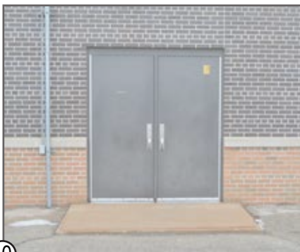
⑩ HOLLOW METAL DOORS & HOLLOW METAL FRAME
